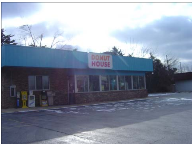
The Donut House is another vacant business along Lincoln Trail .
