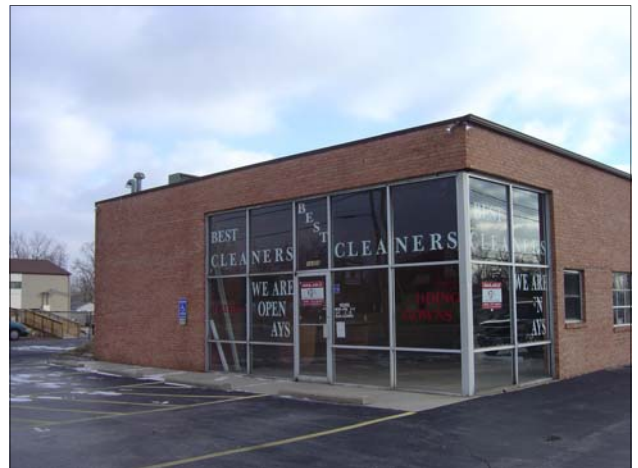
Best Cleaners is a vacant commercial building along Lincoln Trail.
