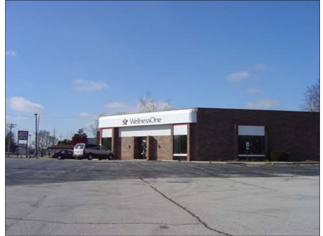
The parking lot for the WellnessOne is cracked and crumbling.
