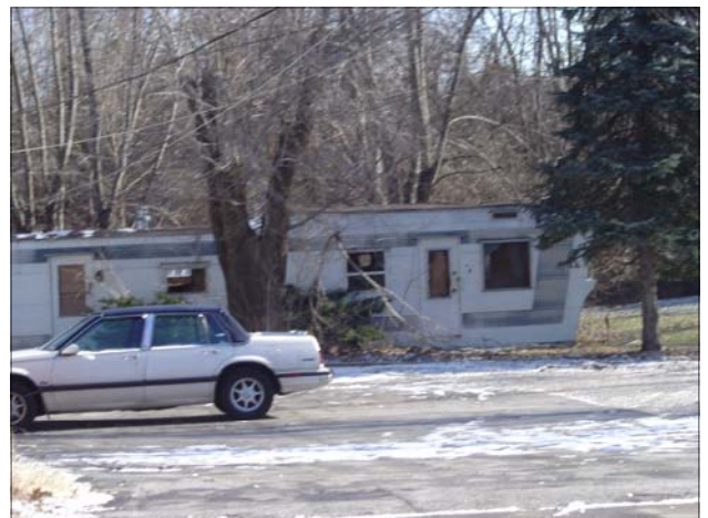
One of the mobile homes fronting Ruby is sitting vacant and deteriorated.
