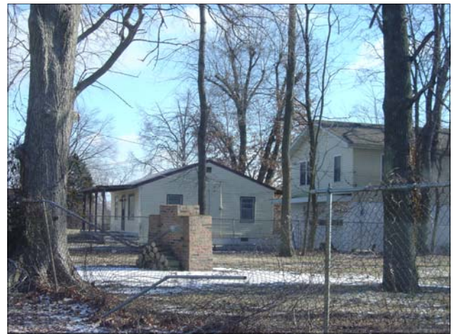
The fence is falling down in front of one of the single-family homes fronting Pasadena.
